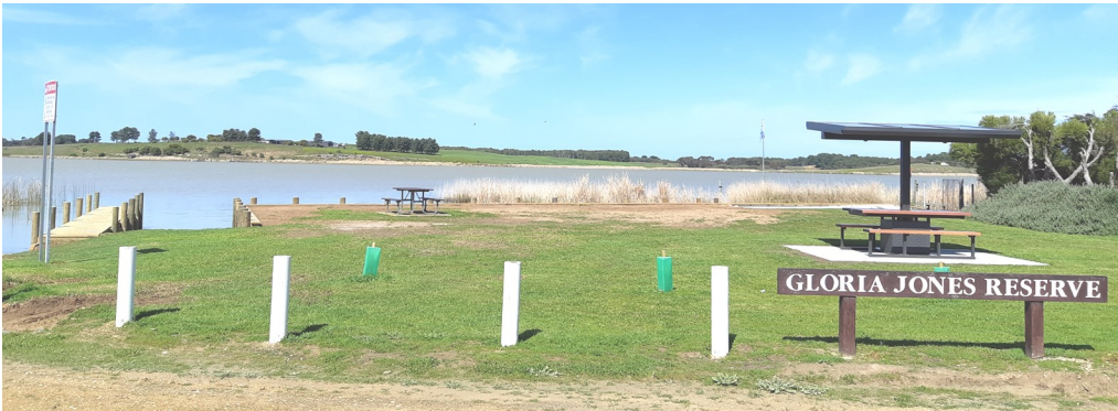
Above: The Gloria Jones Reserve, Rankine Street, now has a smart shelter, new jetty and retaining wall.
