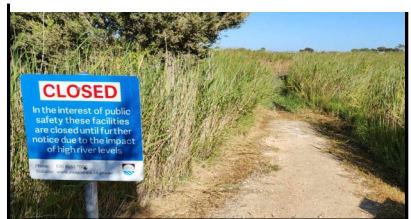
Below: The boardwalk is closed for repairs.
